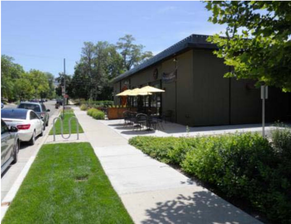
Building front with outdoor patio and bike rack
